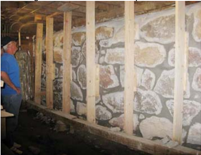
Board member Jim Olsen looks over new foundation
